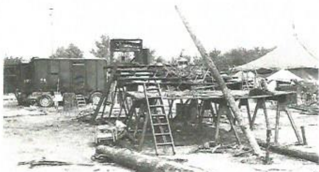
Ringling Band bandstand in Hartford after the fire
